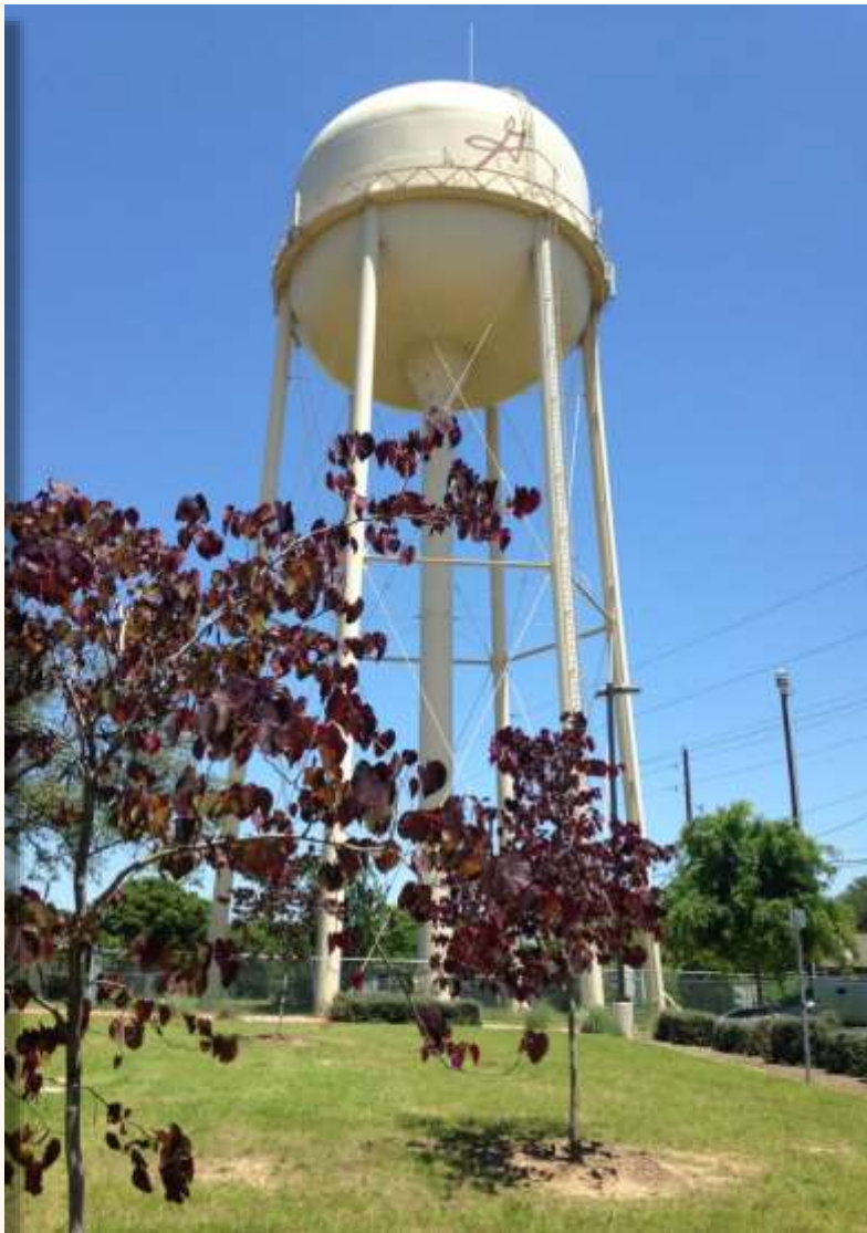
City Elevated Storage Tank
