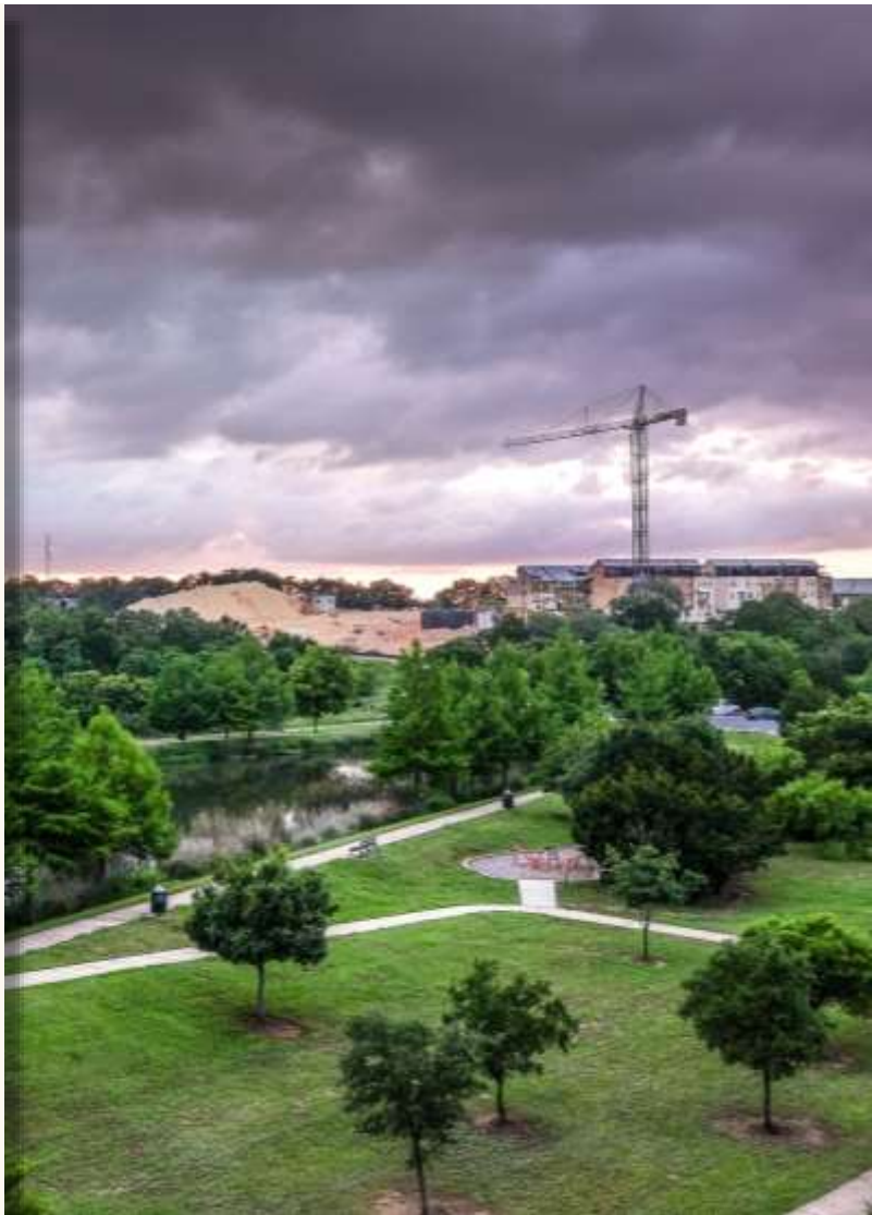
Sheraton Hotel and Conference Center under construction
