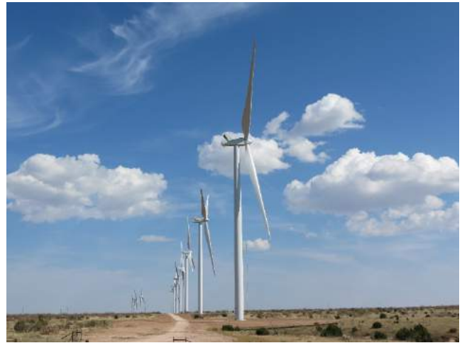
Spinning Spur 3 Wind Farm
