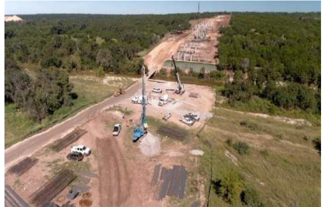
Construction of the Southwest Bypass
